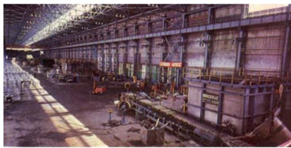
Inside one of the factories of the aluminum plant in Tursunzoda
